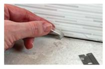
Cut away and remove all caulk with a caulk remover tool or razor blade.
