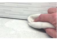
4. Thoroughly wipe down the area with Acetone or Isopropyl Alcohol to remove any silicone residue or sealant that is left behind.
