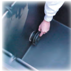
Install fitting with rubber gasket on the inside and the nut on the outside.
