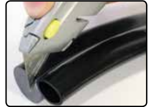
Figure 2. Be careful not to damage the bubble tubing when splitting the ends away from the ballast.
