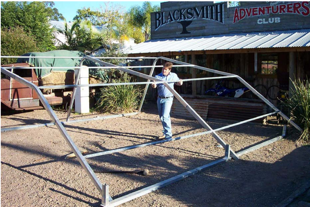
INSERT THE SUB FRAME (NO LADDER REQUIRED)
