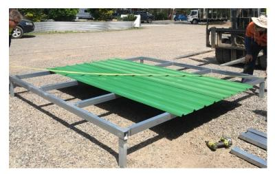
5. Screw cross members to the main frames, using 2 screws per side (offset diagonally)
