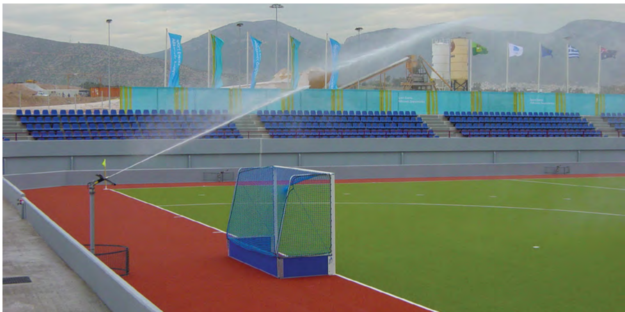
Figure 29. Permanent solid set Big Gun® sprinklers irrigate synthetic turf at the Olympic field hockey stadium in Athens, Greece.
