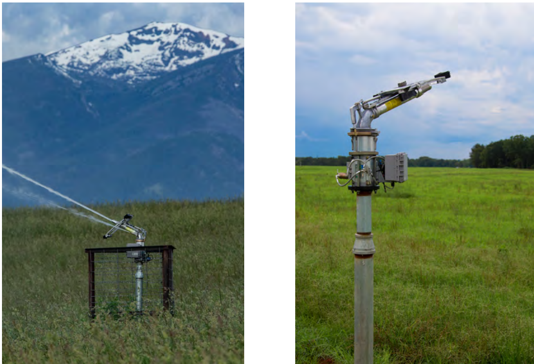
Figure 17. Protect risers from livestock by using a fence (left) or tall risers (right).
