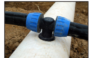
DRIPLINE SECURED TO THE TEE START CONNECTOR
