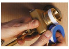
4. Thread tape - Apply PTFE thread tape or approved sealant to the inlet thread and screw the valve into the tank/trough outlet.
