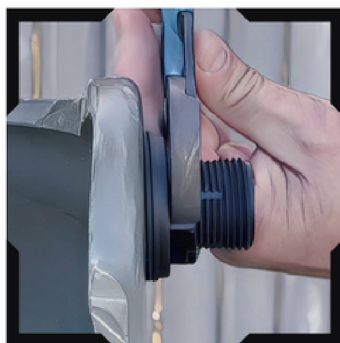
5 TIGHTEN WITH A WRENCH TO ENSURE SECURE SEAL
