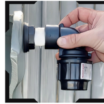
6 APPLY THREAD TAPE AND INSTALL PLASSON FITTINGS
