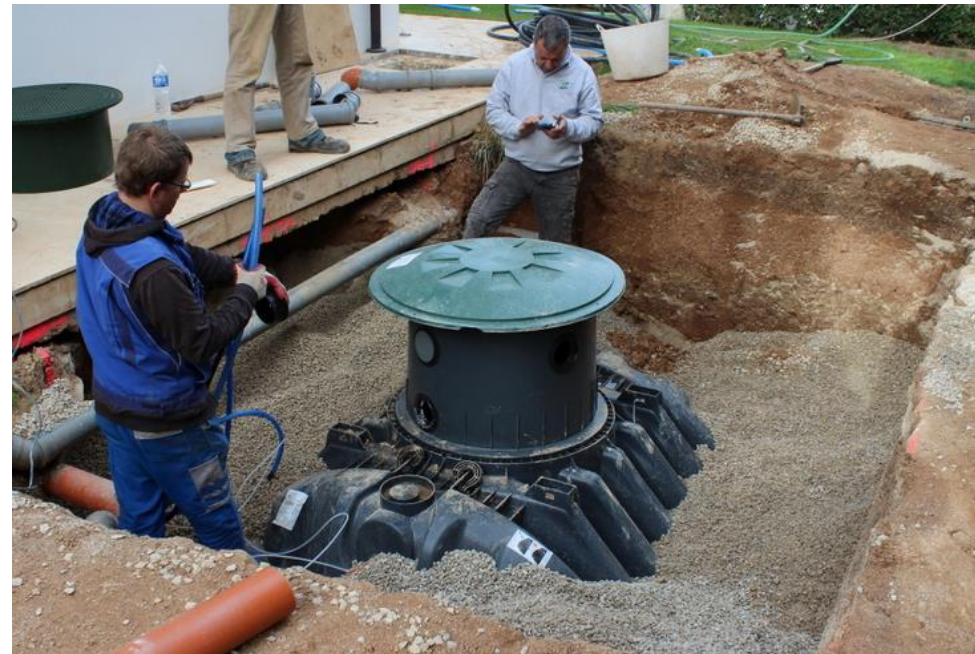
Correct backfill
