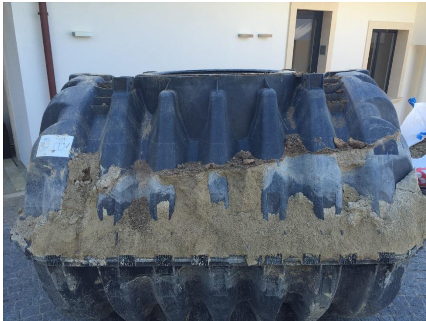
Wrong backfill
