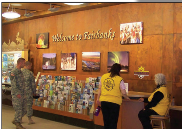
Left: Japanese Brown and Ferric Nitrate applied to steel panels at the Fairbanks Alaska Airport.
