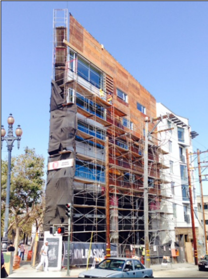
2175 Market San Francisco - Aluminum panels coated with Iron B Metal Coating and rusted with Light Green Patina.
