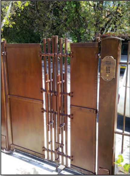
Right: Japanese Brown applied cold on cold rolled steel. Sealed with Ever Clear. Patina by Israel Garcia.
