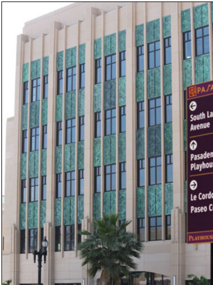
Pasadena Playhouse - Fiberglass panels coated with special mix Darkened Bronze B Metal Coating and aged with Original Blue Patina.
