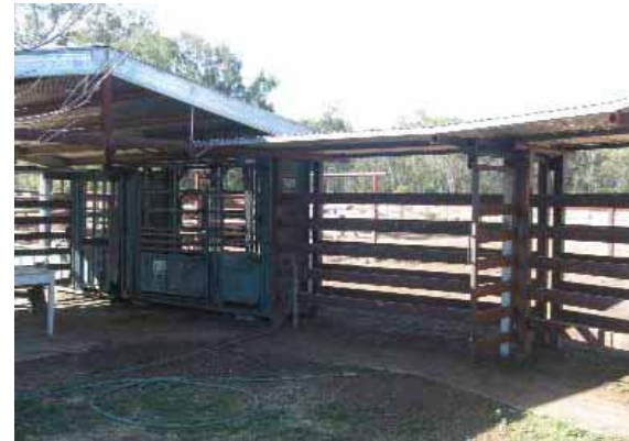
A roof over the working area gives protection from sun and rain.
