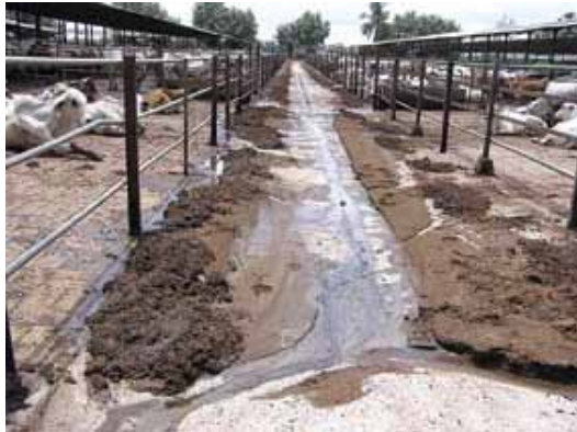
Posts without concrete collars will rust at ground level.
