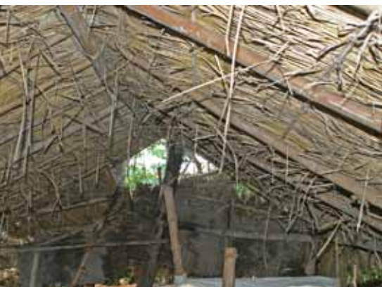
A roof from local materials is cheaper to erect and provides better insulation than tin or tiles, but will need to be replaced periodically.
