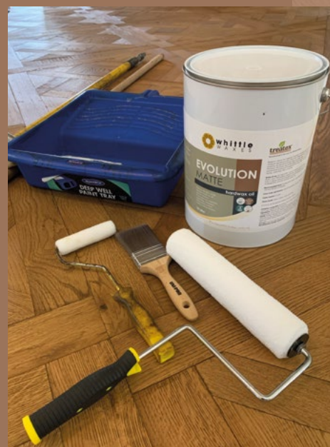
Applying hardwax oil with a roller.
