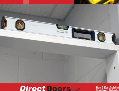
Stand the frame in the new opening and using a spirit level make sure the lintel is level, now check each leg is level on both surfaces (edge and face).
