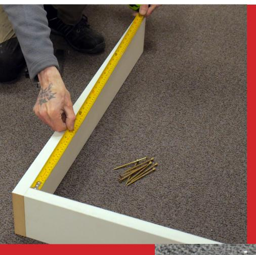
Firstly, measure the opening you have and confirm that the frame kit and door size you intend to use will fit. Please refer to the table above for the overall width of the frame including clearances.
