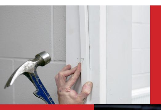
Pin the lintel into position to suit the door thickness, now do the same with the door stop legs.
