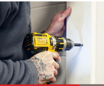
Pre-drill and countersink the legs as and where you deem fit but try and hide some of these screw fixing holes behind the supplied MDF door stops - it's more professional and tidier.
