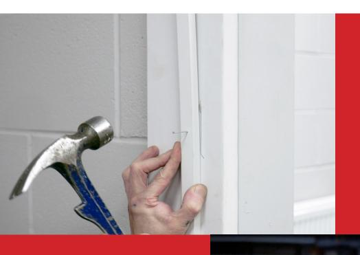
Pin the lintel door stop into position to suit the door thickness, now do the same with the door stop legs. For fire doors, the stops must be screw fixed.
