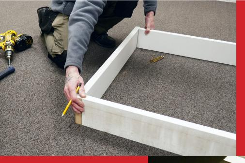
Next, lay each frame leg and the lintel on the floor or on a bench.
