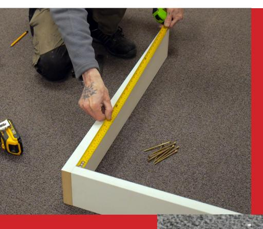
Firstly, measure the opening you have and confirm that the frame kit and door size you intend to use will fit. Please refer to the table above for the overall width of the frame including clearances.
