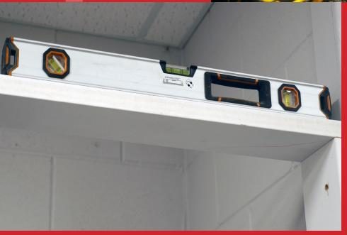
Stand the frame in the new opening and using a spirit level make sure the lintel is level, now check each leg is level on both surfaces (edge and face).
