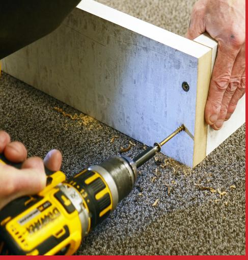
We supply the lintol pre-drilled at one end to match where both frame legs have also been predrilled. We cannot predrill the lintol at one of the ends as we do not know your door size or the clearances you will use, we however, supplied a small predrilled offcut to help you drill in the correct position to suit the predrilled legs, just place the template flush with the frame leg edge and drill through.
