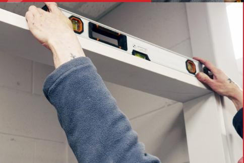
Continue to check the frame is square and level as you proceed with fixing these screws to the top of your wall.
