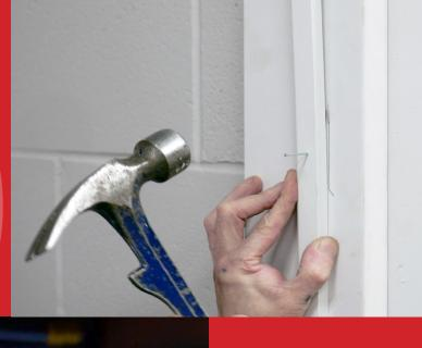
Lastly, fill in any pin holes on non fire frame door stops.
