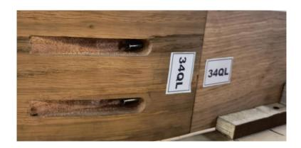
Once all 4 screws are in loosely, tighten all 4 screws one by one until the frame jamb is connected tightly and firmly to the curved frame top. Make adjustments where needed to ensure the vertical frame jambs are fitted flush with the curved frame head on all four edges.
