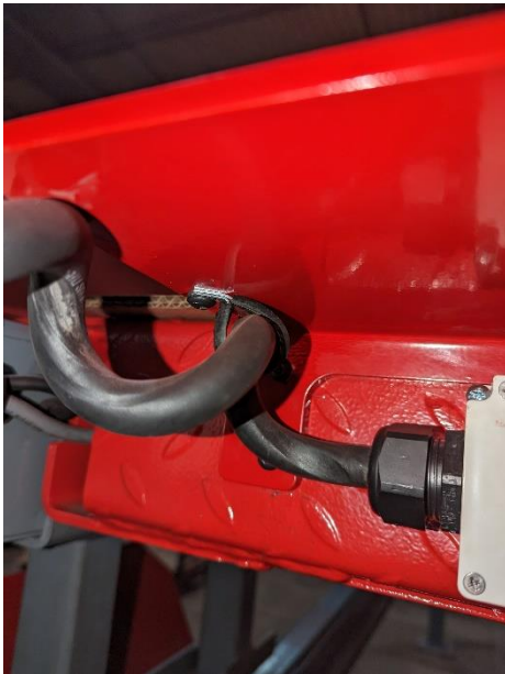
Picture 4.1 Cable pulled slightly tight through loop holder, Top runway.
