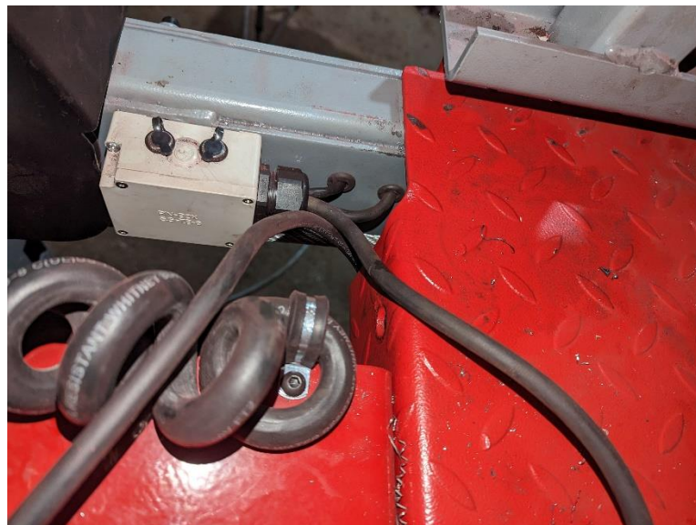
Picture 4.2 Cable pulled slightly tight through loop holder, bottom runway.
