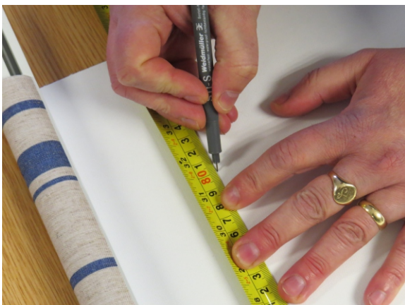
Step 7a. Marking the desired blind width
