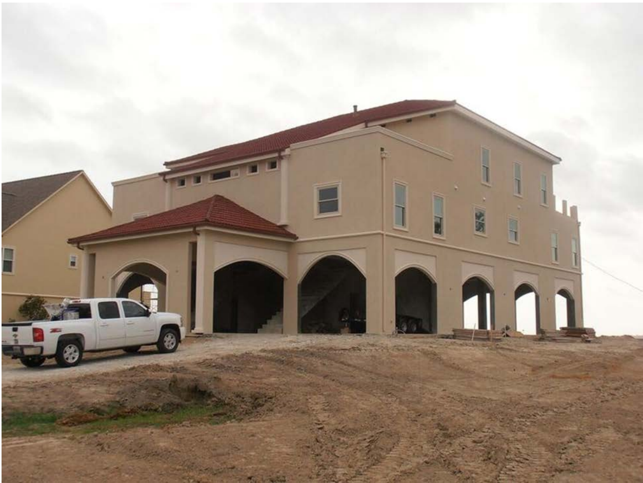
(Photo courtesy of and by permission of Gulf Concrete Technology, Long Beach, Mississippi USA)
