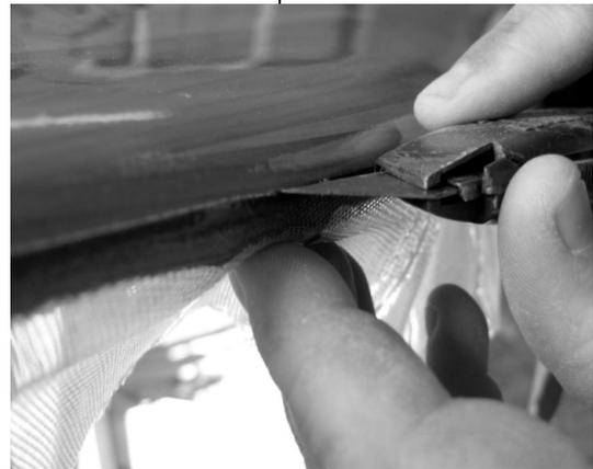
**FIGURE 2-14.** Trim the tape (and glass if any) carefully. Don't cut into the board beneath.
