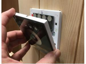
Snap the glass panel onto the control by aligning the notches on the bottom of the panel first then pivoting the glass panel horizontal. Use light pressure to "snap" the glass cover in place.
