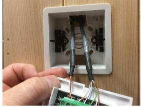
Insert the two CAT5 cable ends into the upper or lower opening in your enclosure. (upper will allow more cable to be in the wall)
