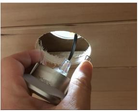
Using a drill-mounted hole saw, cut a 2 ¾" hole at each of the desired locations in your ceiling. Carefully compress the two spring clips on the fixture and insert them into the hole until they are past the thickness of the ceiling material. Slowly allow the clips to pull the fixture up into the hole to secure it to the ceiling.
