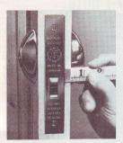
PICTURE 25 Measure distance from outside of door to edge of forend.
