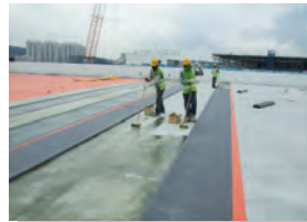
2) Laying of Root-proof Waterproofing Membrane.
