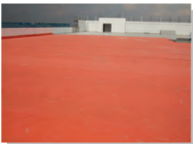
3) Completed waterproofing membrane.
