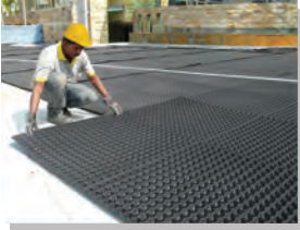
3) Properly aligning of PlanterCell® 30 Green Roof trays.
