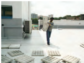
3) Marking out and setting out of Insu® Slab onto prepared surface.
