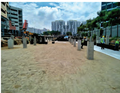
2) Laying and levelling of sand layer.
