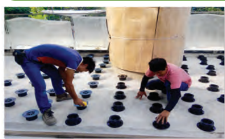
1) Setting out pre-assembled Insu® Jac pedestals
