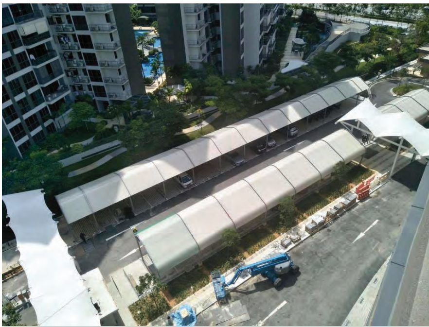
Project: Detention Tank, Global Indian International School Carpark, Punggol, Singapore
