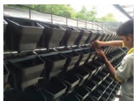
2) Installation of Auto-Irrigation lines.
