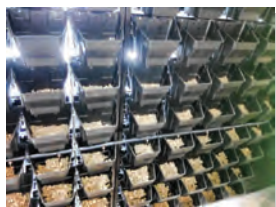
4) Laying of PlanterCell® Planting Mix.
