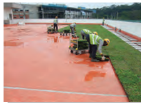
4) Laying of pre-planted PlanterCell® 70 Green Roof trays.
