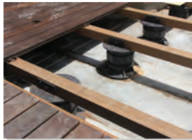
5) Installation of timber board decking.
