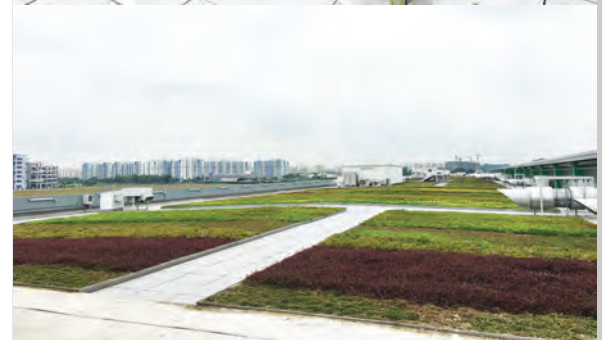
Project: Bulim Bus Depot, Singapore
