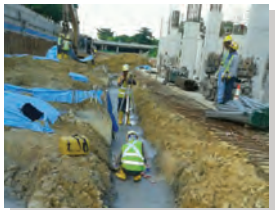
1) Levelling of surface according to design gradient.
