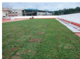
6) Completed Green Roof.
