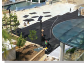
2) Laying of PlanterCell® 30 Green Roof trays.
