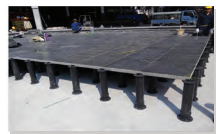
3) Installing granite slabs
