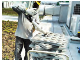
4) Applying PU grout at the bottom for spot-bonding.
