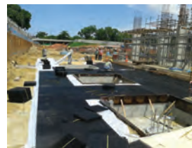
9) Laying of Insu® Felt and DC30 Drainage Cell.
