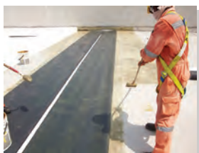
3) Application of bonding adhesive.
