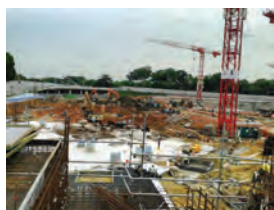
8) Levelling of soil surface at sub-basement level.
