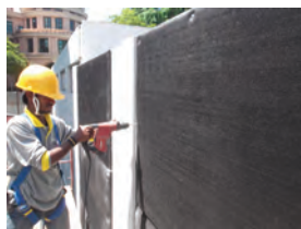
2) Setting-out & fixing of panels onto the prepared wall surface.
