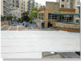
1) Laying of Root-proof Waterproofing Membrane.
