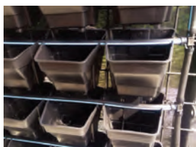
3) Connection of Auto-Irrigation lines.
