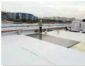
1) Installation of waterproofing membrane.
