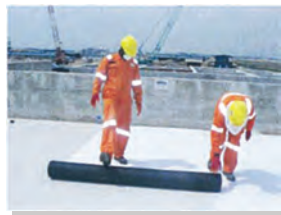
2) Unrolling of PVC membrane over prepared substrate.
