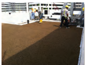
5) Installation of geotextile, planting media and plants.
