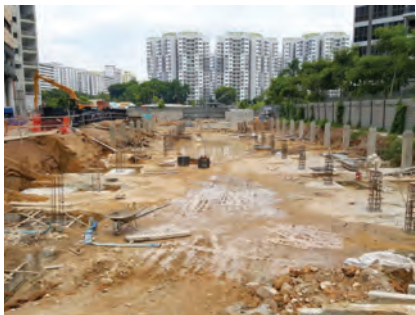
1) Excavation and preparation of lean concrete base as per PE specifications.
