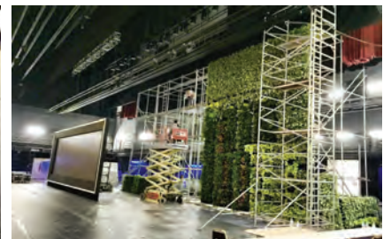
6) Setting-up and installation of the P.E. approved scaffold frame.
