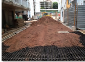
5) Laying of soil.
