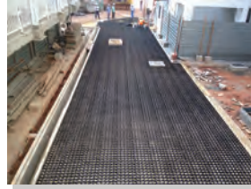
4) Prepared area with levelled GrasCell® GP40.
