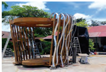
4) Installation of greenwall panels for the Garden Shed feature.
