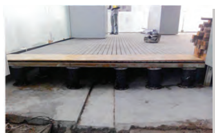
5) Installation of bamboo decking
