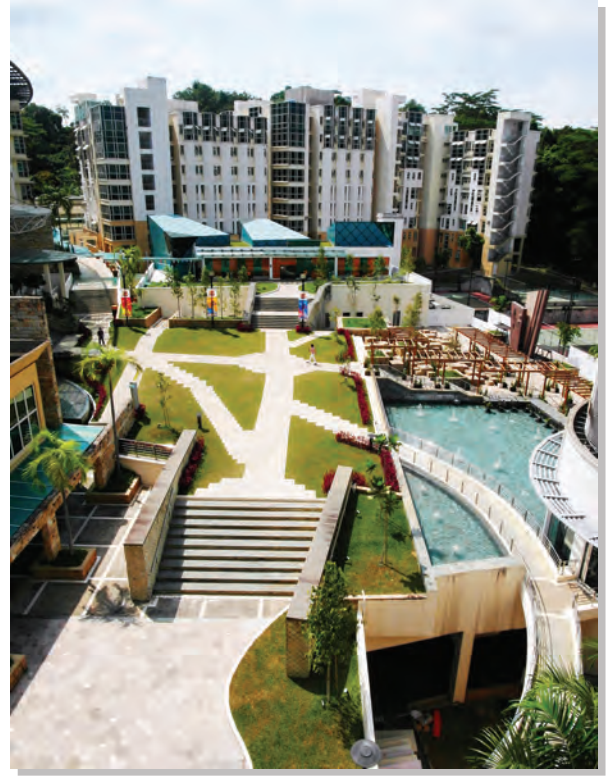
Project: Prince George's Park Residence - NUS, Singapore
