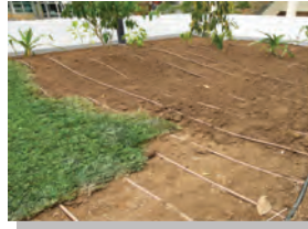
6) Laying of Auto-Irrigation lines and ground cover plants.
