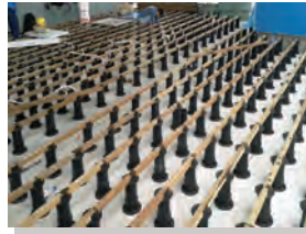
3) Installation of wood battens and bearers.
