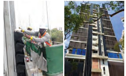
3) Installation of PlanterCell® 170 greenwall trays.
