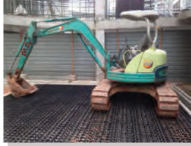
3) Compacting and leveling of surface.
