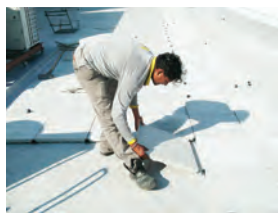
6) Securing the Insu® Slab onto the prepared surface.
