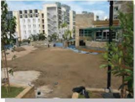
5) Laying of PlanteCell® Planting Mix.
