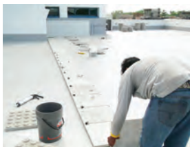
5) Installation of Insu® Slab spacers.
