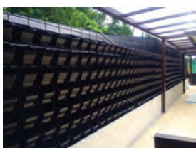
1) installation of PlanterCell® 170 Mini Green Wall trays.
