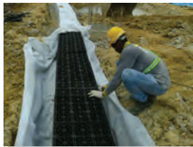
5) Cover SW Tank with Insu® Felt prior back fill.
