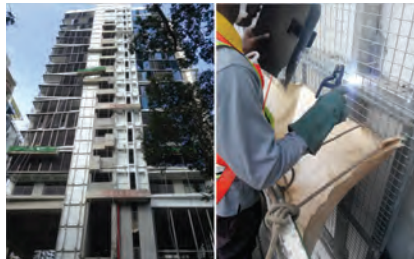
2) Installation of main frames at site.
