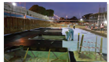
10) Installing Insu® Felt over DC30.
