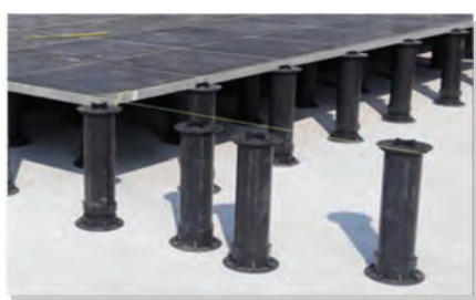
1) Setting out pre-assembled Insu® Jac pedestals
