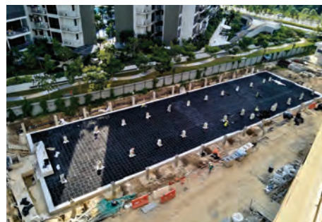
6) Subsequent laying of the PlanterCell® SW Tank.
