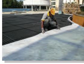
4) Laying of 120g/m 2 Insu®Felt geo-textile.
