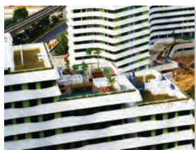
6) Completed greenroof with Root-shield waterproofing membrane.
