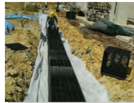
3) Installation of SW Tank.
