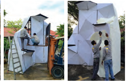
3) Setting out of the greenwall panels to form the Waterfall feature.
