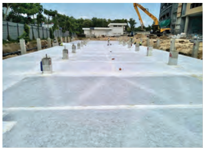
7) Completed Insu® Felt geotextile on top of detention tank.
