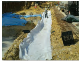
2) Laying of Insu® Felt over proper prepare surface.
