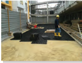
1) Laying of GrasCell® GP40 onto the prepared leveling sand.
