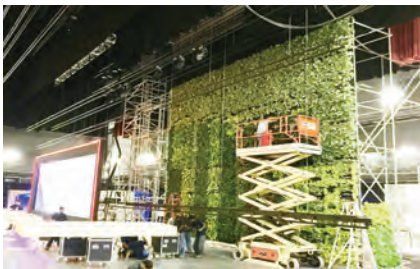
7) Installation of greenwall panels onto the completed scaffold frame.
