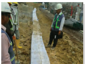
7) Completion of back filling.
