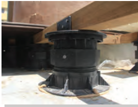
4) Securing the wood battens onto the Insu® Jac pedestal.
