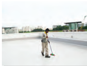
2) Surface preparation and cleaning prior to installation of Insu® Slab.
