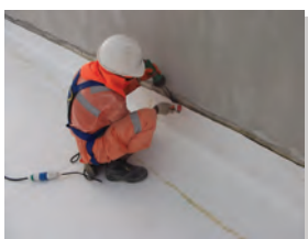
5) Grooveline tuck-in for upturn and detailing areas.
