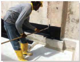
3) Upturn and corner detailing.
