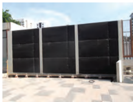
3) Completed installed panels.
