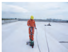
4) Hot welding of over lapping joints and edges.
