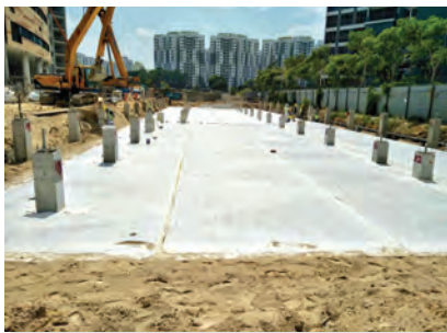
8) The perimeter is filled with sand to aid in filtering the water draining out at the sides of the tank.
