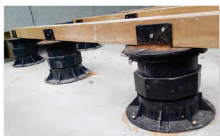
4) Secure wood battens onto Insu® Jac Wood Holder using screws
