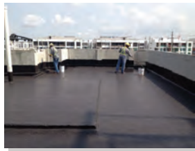
4) Whole roof area coverage.
