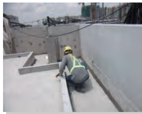
2) Installation of angle fillets.
