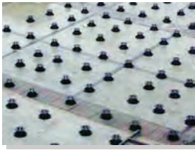
1) Setting out of Insu® Jac pedestals.
