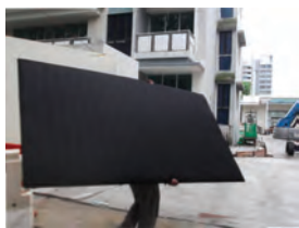
1) Pre-packed panels are delivered at site.
