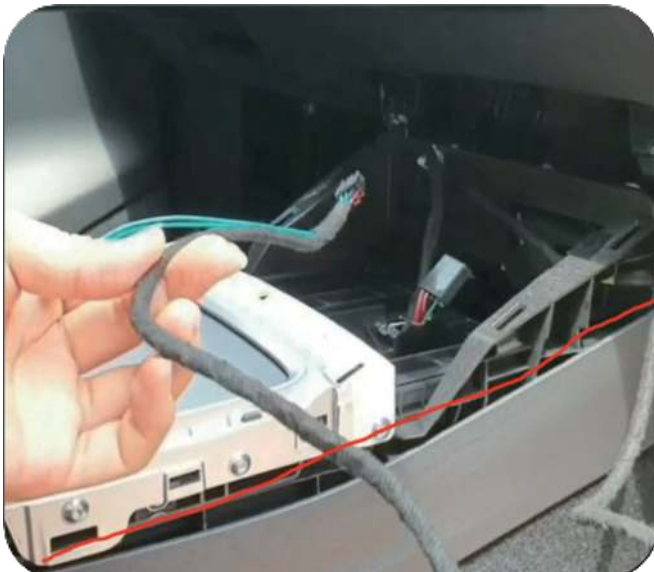
11. Lead the wiring from the lower cover panel to the center console
