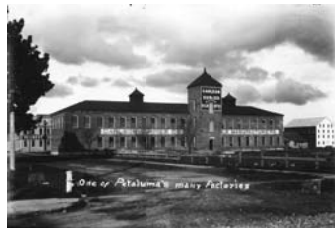
VIEW OF ORIGINAL 1892 SILK MILL BUILDING
