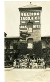
VIEW OF STAIR TOWER #1
