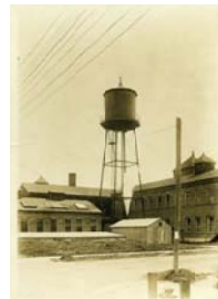
VIEW OF WATER TOWER
