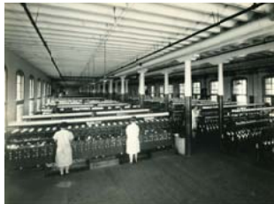
VIEW OF FIRST FLOOR MILL OPERATIONS
