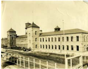
VIEW OF 1922 SILK MILL BUILDING
