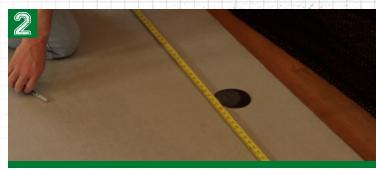
Fold the rubber tee in half, feeding it through the hole. If at first it doesn't fit, take the drill and expand the hole a little more, making sure it's still a nice and snug fit. You have now successfully installed the rubber tee.
