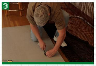
Use the black marker to trace the template; with the utility knife carefully cut out the hole.
