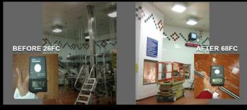
for easy, tool-less access to ballast and wiring. The new AEI Lighting system reduced the lighting load from 465 Watts per unit to 234 Watts per unit. AEI's design and interior architecture solution also doubled the existing foot candles, and now provides instant on and instant restrike after power interruption. With the higher CRI and consistent color from fixture to fixture, Ralph's management considers the lighting project a major success.
