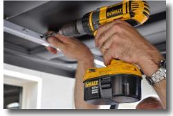
Attach mirror bracket to roof strut using included self tapping screws. *Tighten completely.*
