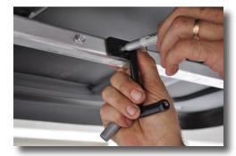
Drill holes into horizontal strut using a 3/16" bit.
