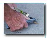
5. Gun Slab into the crack. For wider cracks (1" wide or more), apply 3 beads: 1 on each side of the crack, and another down the middle. This ensures enough product is in the joint, and makes tooling easier.
