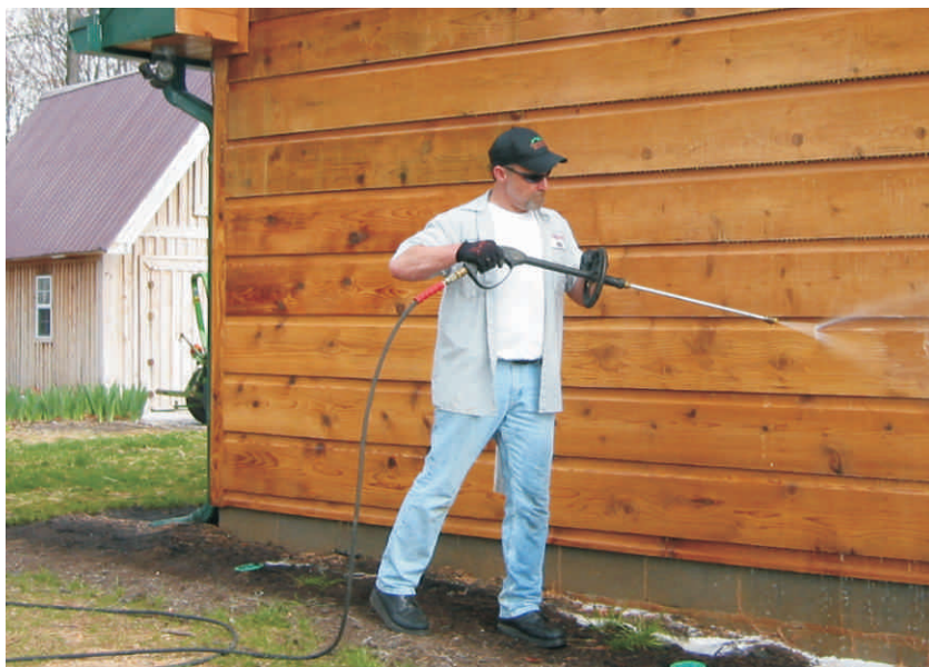
Proper Technique for Pressure Washing
