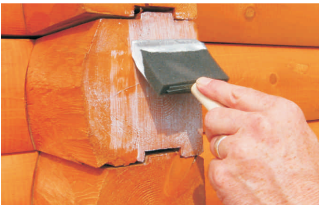
Applying Log End Seal
