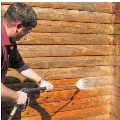
**Step 7:** Pressure wash starting at the bottom of the wall. Work on 2 or 3 courses of logs at a time. Hold the wand at a 30 to 45 degree angle to avoid feathering the wood.
