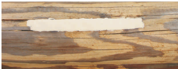
Cavity filled with E-Wood.
