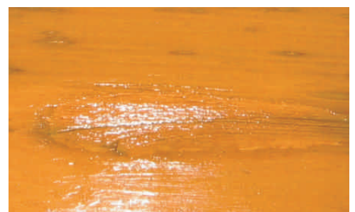
Stained and topcoated.
