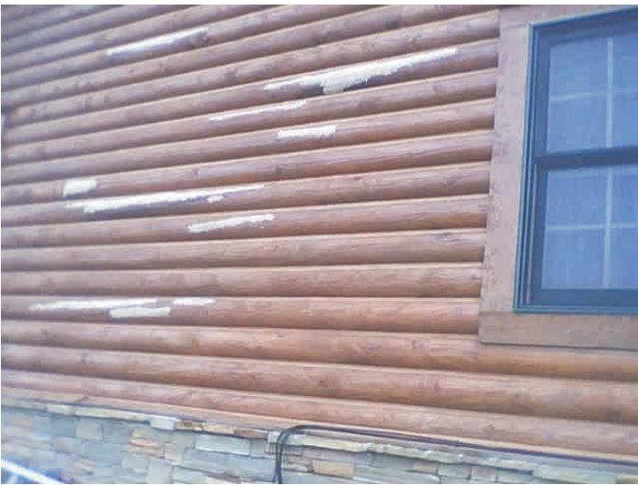
Voids treated with Shell-Guard RTU, M-Balm then filled with 2x4s and E-Wood.
