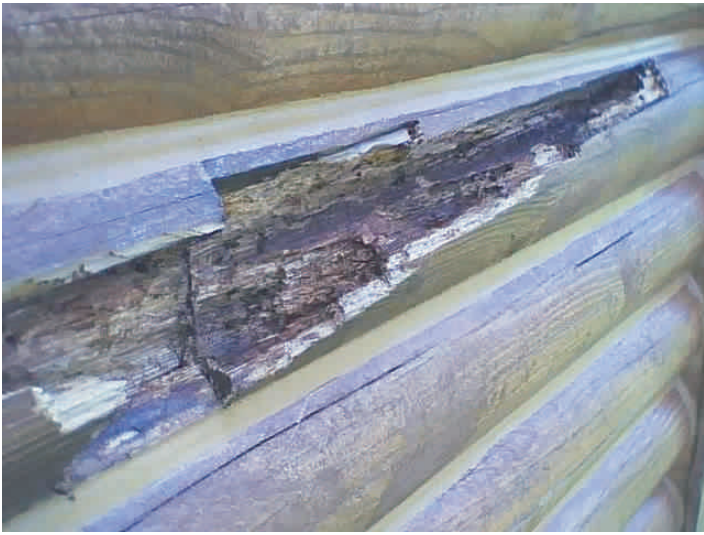
Large voids in logs after removing soft, loose wood fibers.
