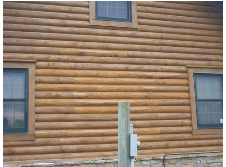
Repaired areas coated with Energy Seal then stained.
