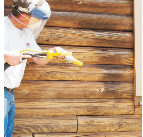
Media blasting with crushed glass
