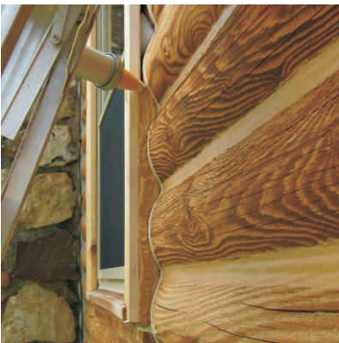
Fill the 3/8" gap between the surface of the foam and the edge of the frame with sealant.
