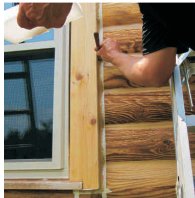
Rough tool sealant into place then lightly spray surface with water and tool smooth.
