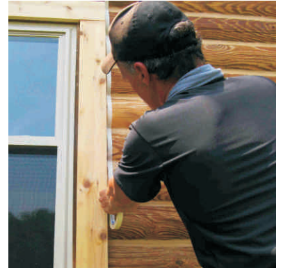
Apply masking tape to prevent sealant from smearing onto the adjacent logs.
