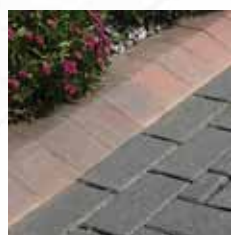
Standard kerb in low position
