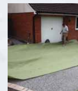
5 Lay Inbitex Geotextile
