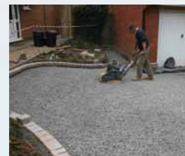
4 Spread and compact 5-20mm clean stone
