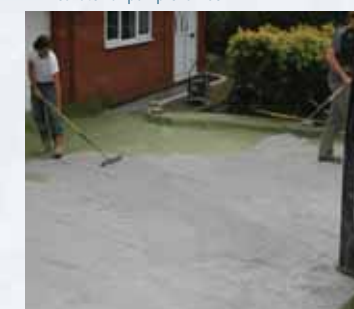
6 Spread and screed 2-6mm clean stone
