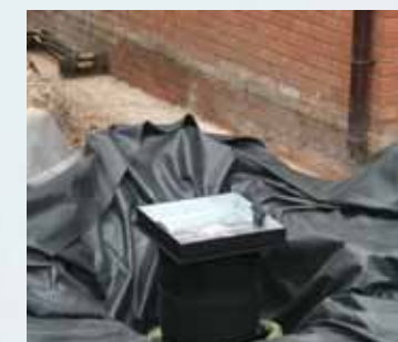
3 Line with impermeable membrane and insert pump
