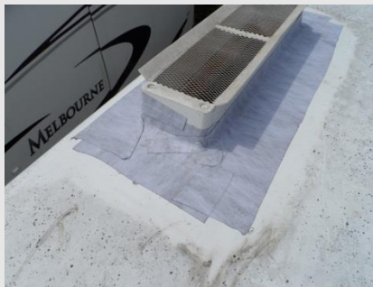
SEAM TAPE APPLICATION
