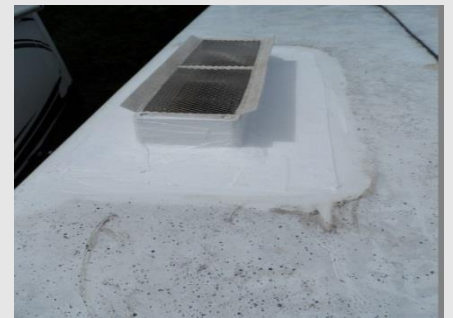
SMOOTH SEALANT APPLICATION
