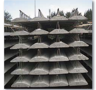
Concrete moulds are made and ready to be laid.
