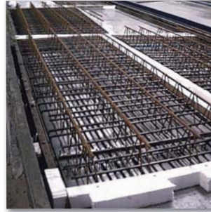
Concrete flooring is sectioned into place.
