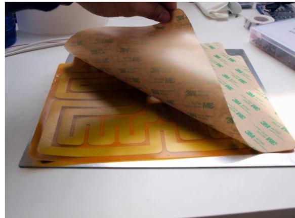
SLOWLY and CAREFULLY remove the protective layer from the foil heater. The adhesive layer should remain intact as good as possible.
