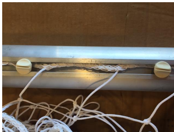
Figure 2. MP Channel Net Fastener in Crossbar tube.
