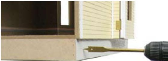
□ 2. If your wiring is already in the cellar, good! Otherwise, drill holes thru the floor to access the house wiring.
