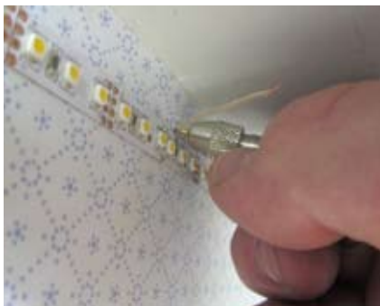
Install a small eyelet in the hole along with the wire.
