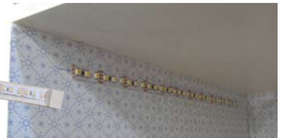
Attach the ExtraBrite® Striplight centered on the 3/4" line
