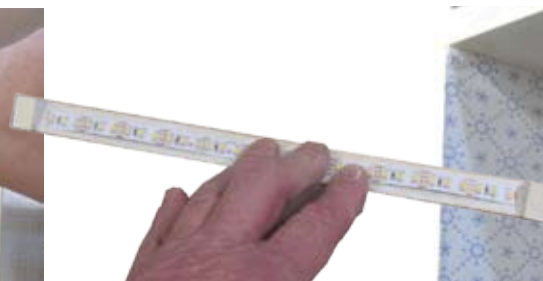
Cut the ExtraBrite® Striplight to fit within the Valance
