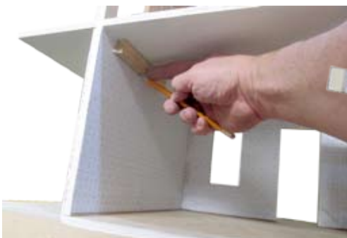
Marking 3/4" below the ceiling
