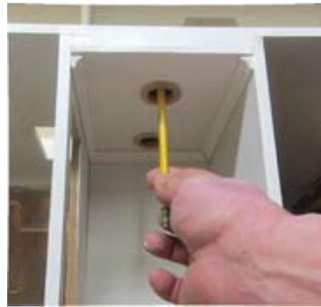
Trace the opening onto the structural ceiling.
