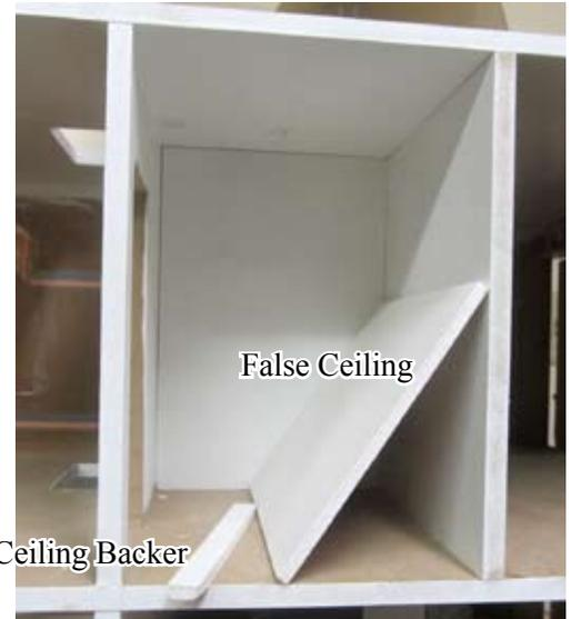
Make a False Ceiling to fit the room in which you will install the recessed light. I am using 1/4" Foamcore Board, but could use 1/8" MDF or Mat Board instead.
