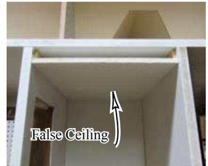
The Stripwood is a spacer for the recess above the False Ceiling.
