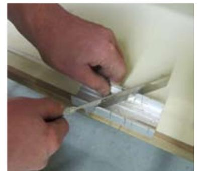
Cut Crown material to fit below the False Ceiling - here I am using crown from the JFK Finishing kit.
