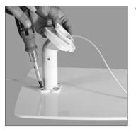
1. Attaching directly to a counter or wall: If you are not using a baseplate and instead attaching your unit directly to a surface you will need to obtain 4 fasteners suitable for your substrate. Use the mount pattern provided on page 6 of this document to mark your screw openings.
