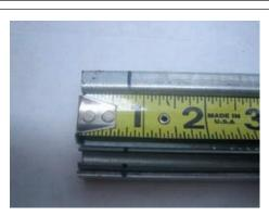
4. On the bottom of the track, mark 3/4 of an inch.
