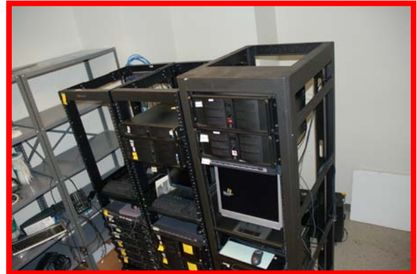
Figure 26. LESS EFFECTIVE – The camera is too close to the area of interest. The camera angle is too sharp and targets would not be in full view (see page 3).
