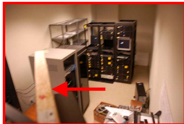
Figure 28. LESS EFFECTIVE – The camera view includes the area where the door will swing open.
